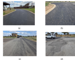
Figure 3. Common Distresses: (a) Longitudinal and Transverse (LT) Cracking. (b) Block Cracking. (c) Weathering and Light Raveling. (d) Localized Patching.
